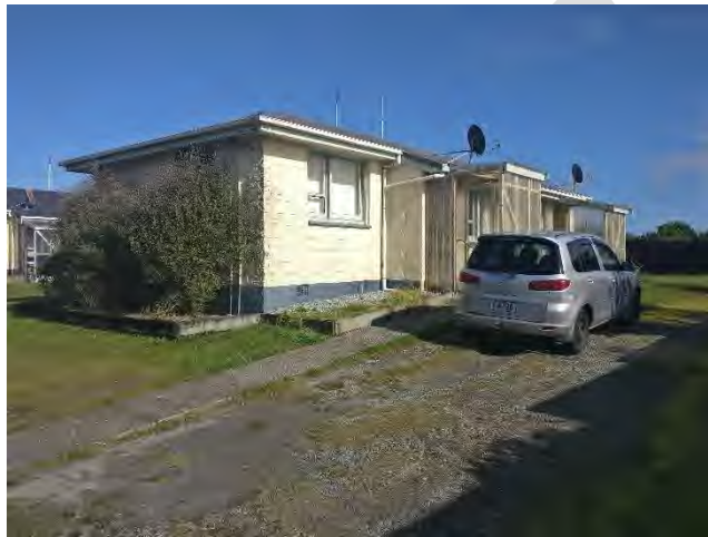
Units at Revell Street
